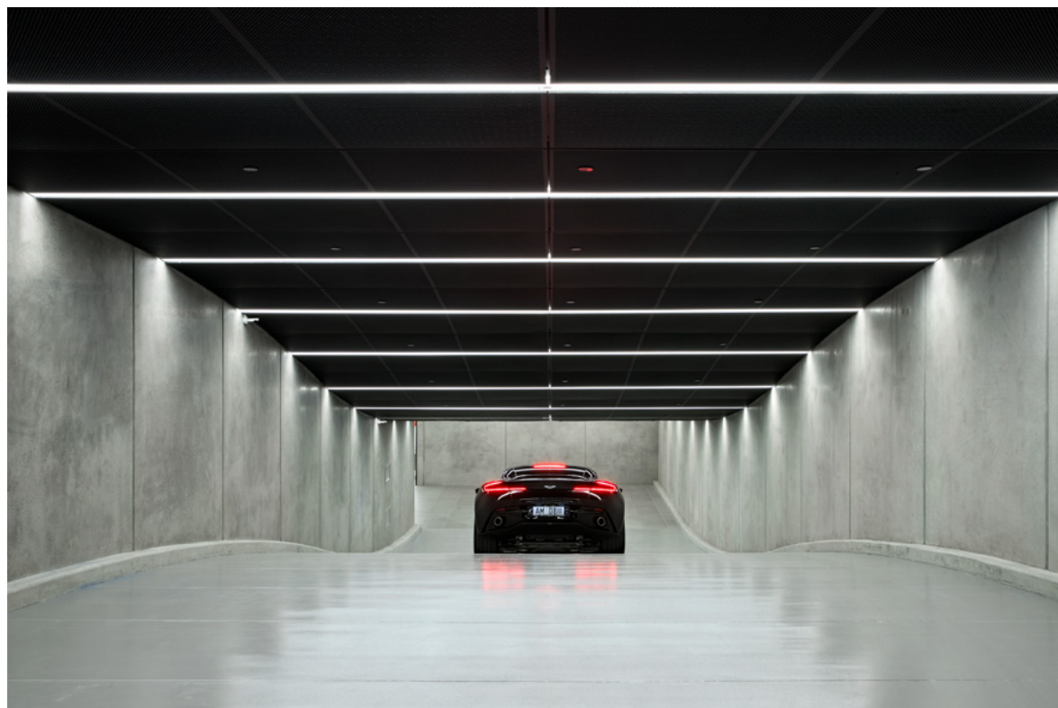
Right A curved ramp, set out to align with a sine wave curve, is designed in order to connect each floor
